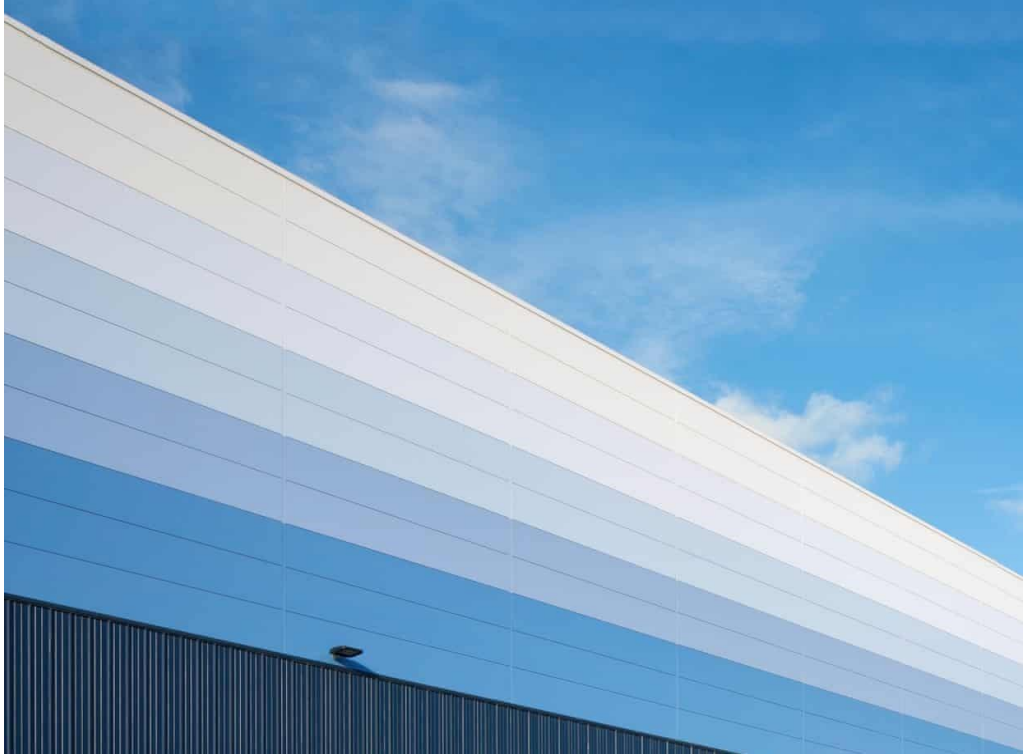
Painting the structure to blend in with the landscape
